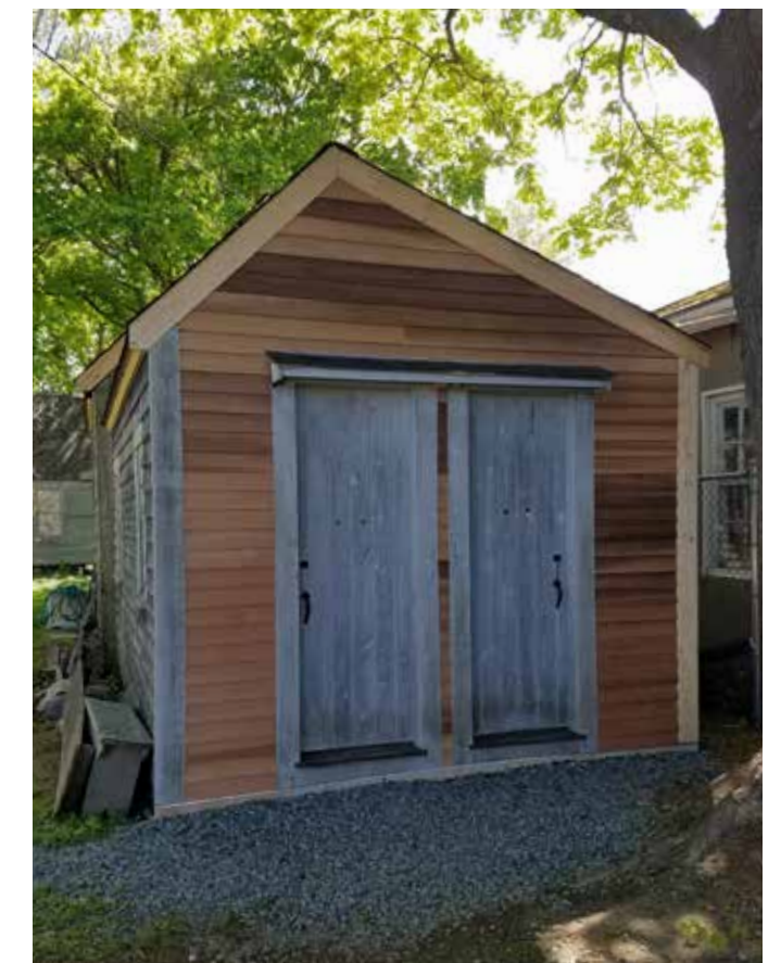
Below: New clapboards on the east end of the bathroom building at the Harlow House, installed by volunteer Karl Lekberg.
